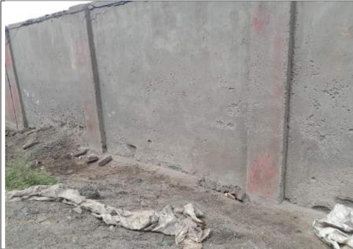
Area near cooling tower is observed dry.
