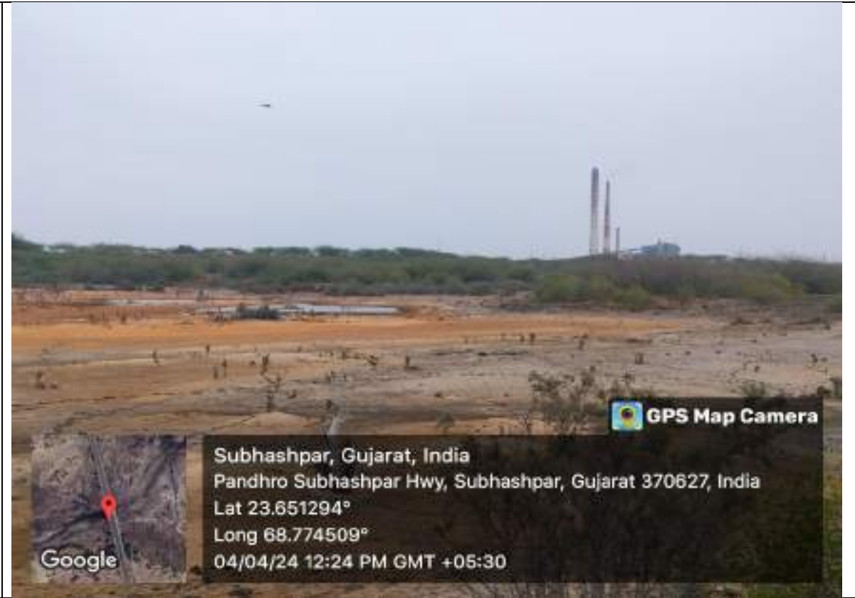
Little water accumulations is observed outside Dyke-C.
