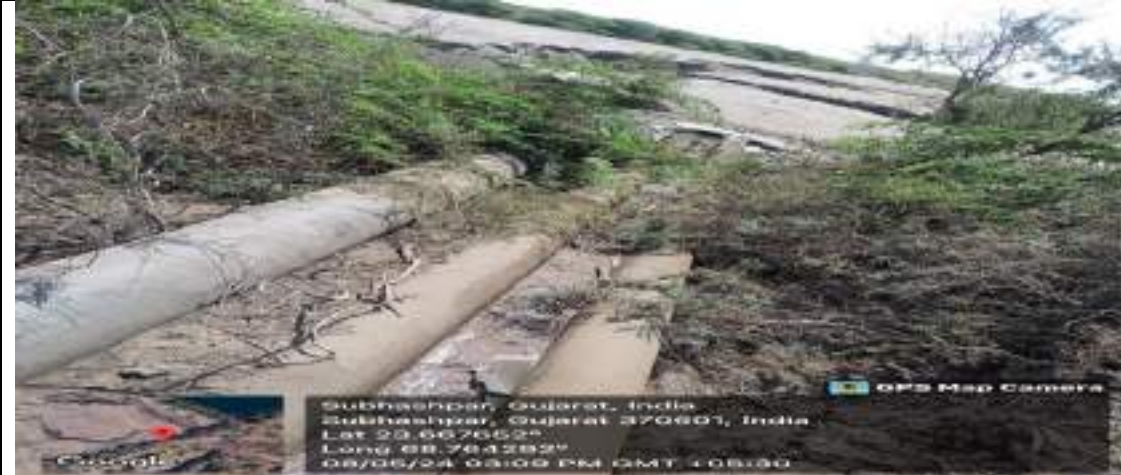
Ash slurry disposing in Dyke-D.
