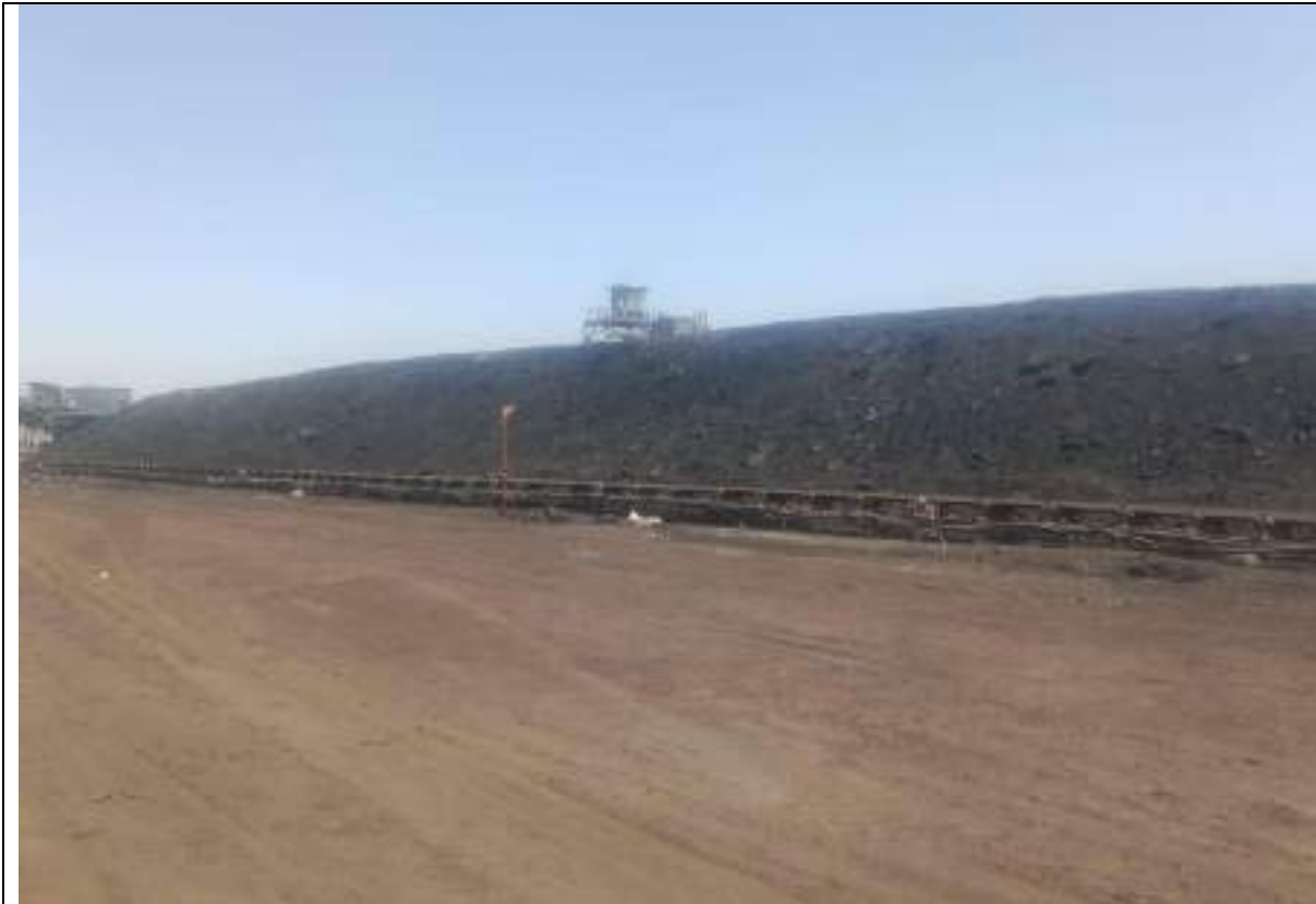
Coal yard with water sprinkling system
