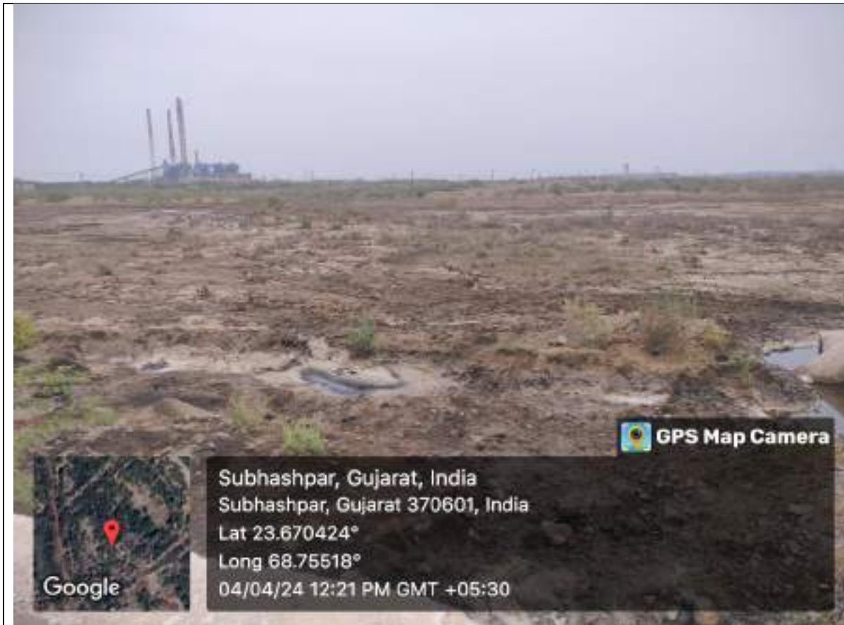
Seepage outside units premises due to Dyke-A.
