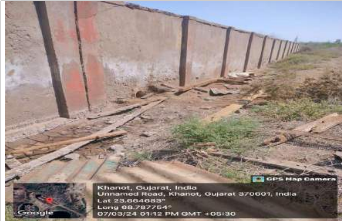
No flow from cooling tower outside unit's premises is observed.
