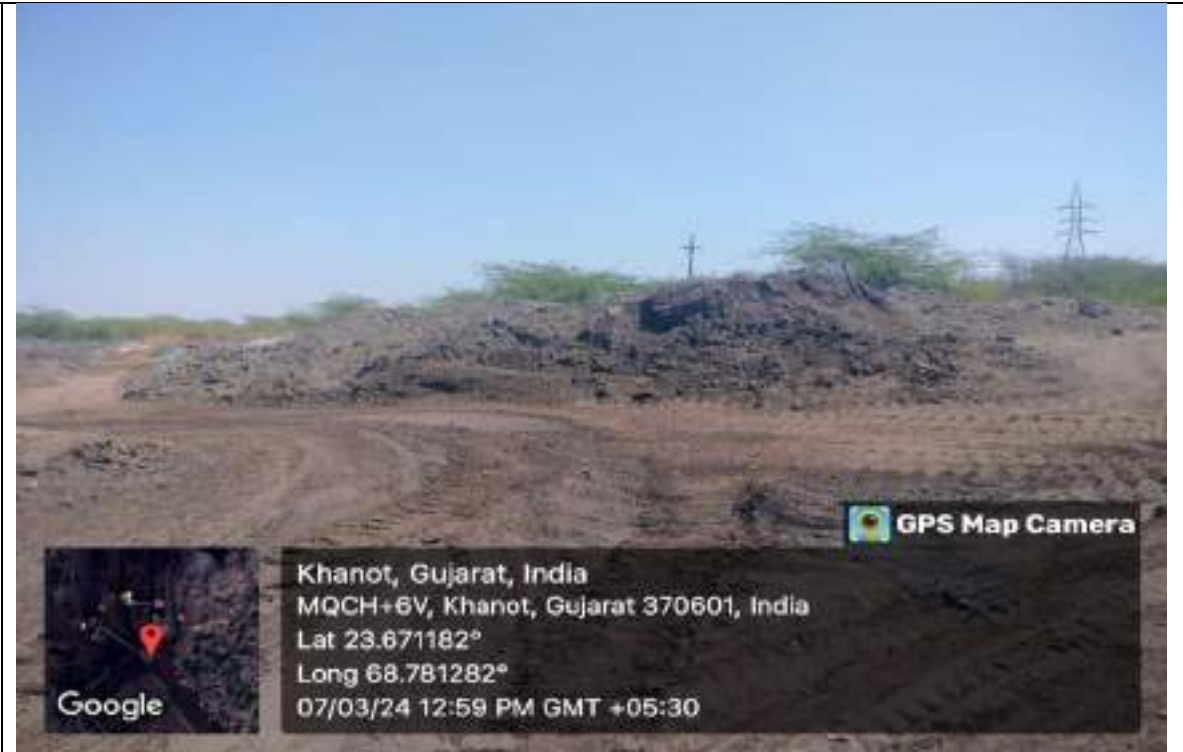
Fly ash dumps near coal yard and outside unit's premises is observed.
