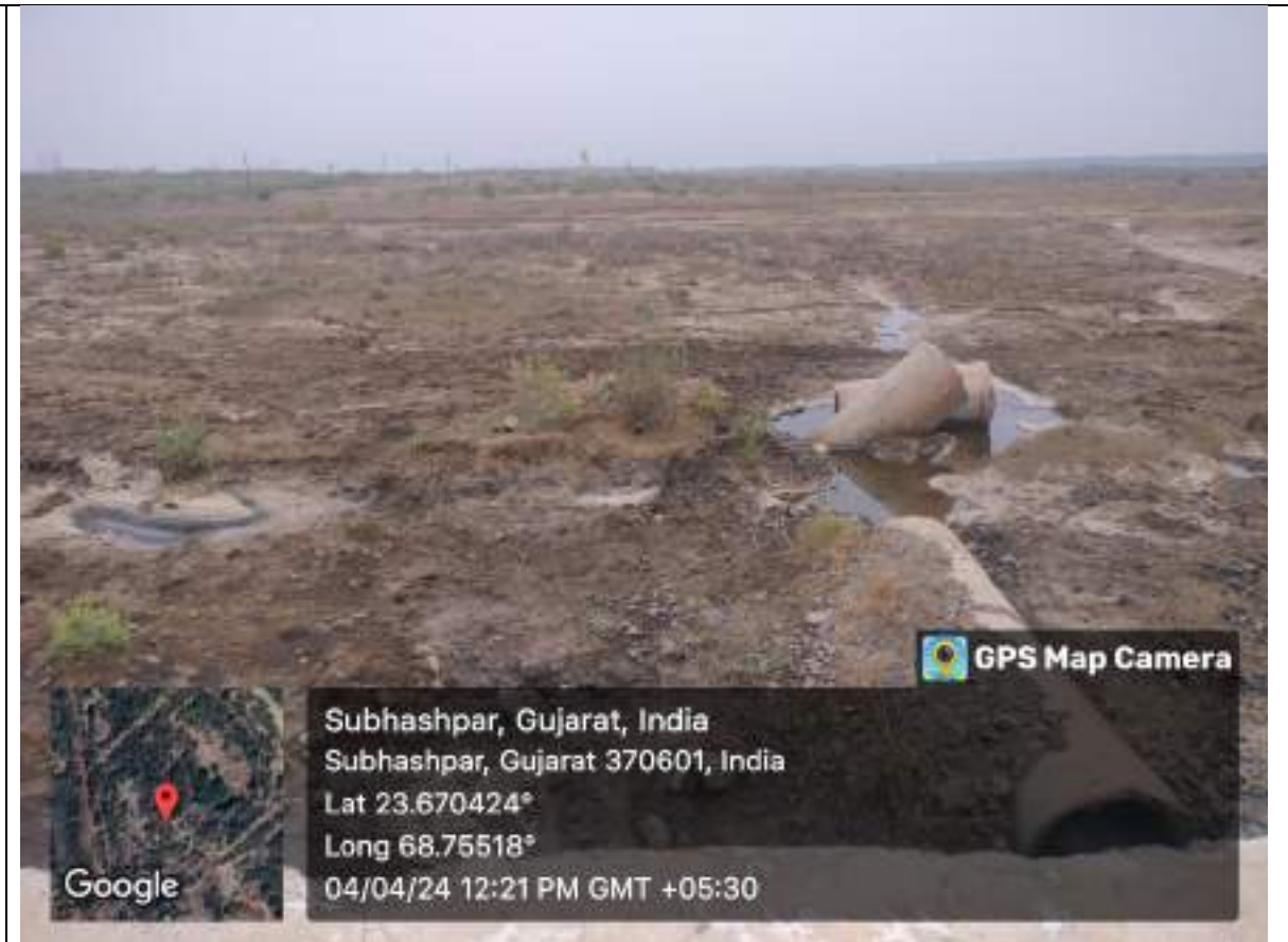
Seepage outside units premises due to Dyke-A.
